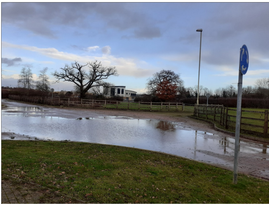
Photo of entrance road (no rain for over 24 hours, Dec 2022)
